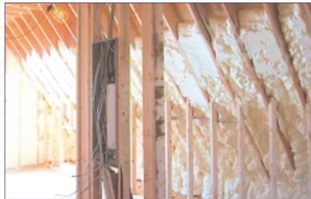
Icynene® was applied to the underside of the vaulted ceiling in the old attic space. This turned the previously unconditioned space into a conditioned living area.
