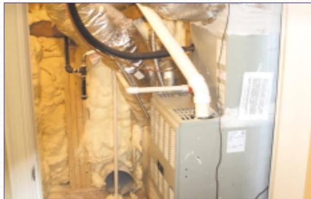
Icynene® was sprayed directly into the wall cavity around the HVAC system and the return and supply ducts. This helped to improve the airtightness of the building envelope and increase the overall energy efficiency.
