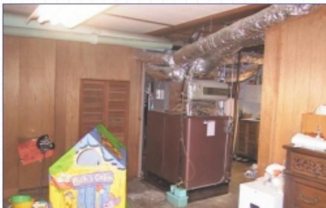
*The original furnace and duct work in the house were circa 1970's. The air infiltration rate was 0.65 ACH (Air Changes per Hour) @ natural pressure. The Icynene® application reduced the rate to 0.37 ACH<sub>nat</sub>.*
